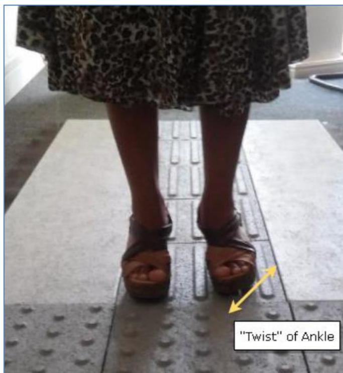
Fig. 11. Twist of Ankle of a Wedge User [8]
