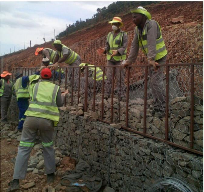
**Photo 3:** Slope stability protection measure on R396 in Tsolo
