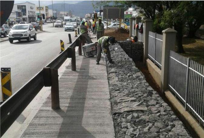
**Photo 2:** A completed walkway and gabion work as a safety measure and erosion protection along the N6 in Queenstown
