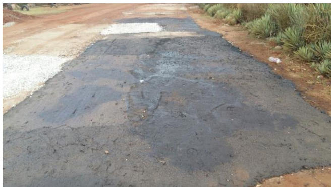
Fig.3 Various DBM test panels with and without penetration slurry for training and evaluation purposes.
