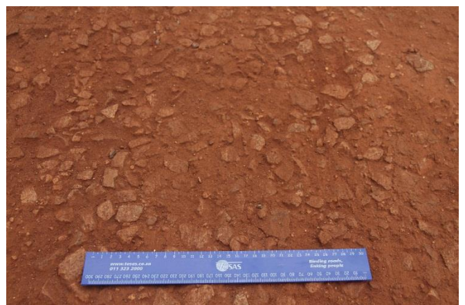
Fig.5 Final coarse aggregate prior to placement of the penetration slurry.
