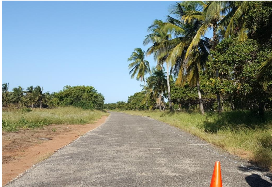
Fig. 5 Penetration macadam section
