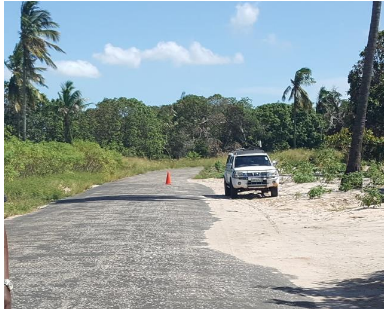
Fig. 7 Sand seal on armoured base section
