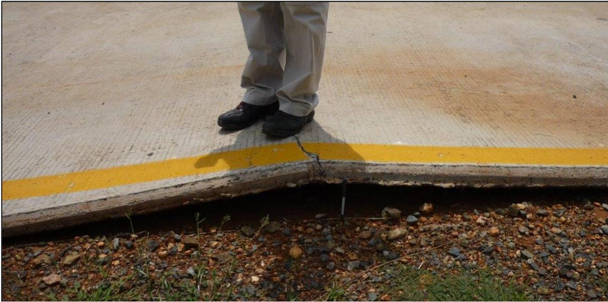
Figure 1: Typical example of a buckling blow-up failure in an ultra thin concrete pavement.
