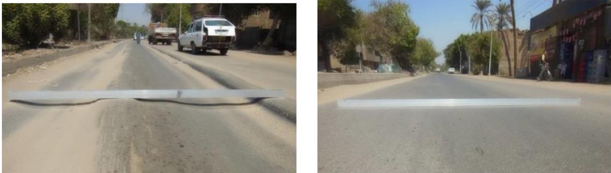
Fig. 7. Rutting depth entities in a unmodified and with Superplast modified asphalt concrete.
