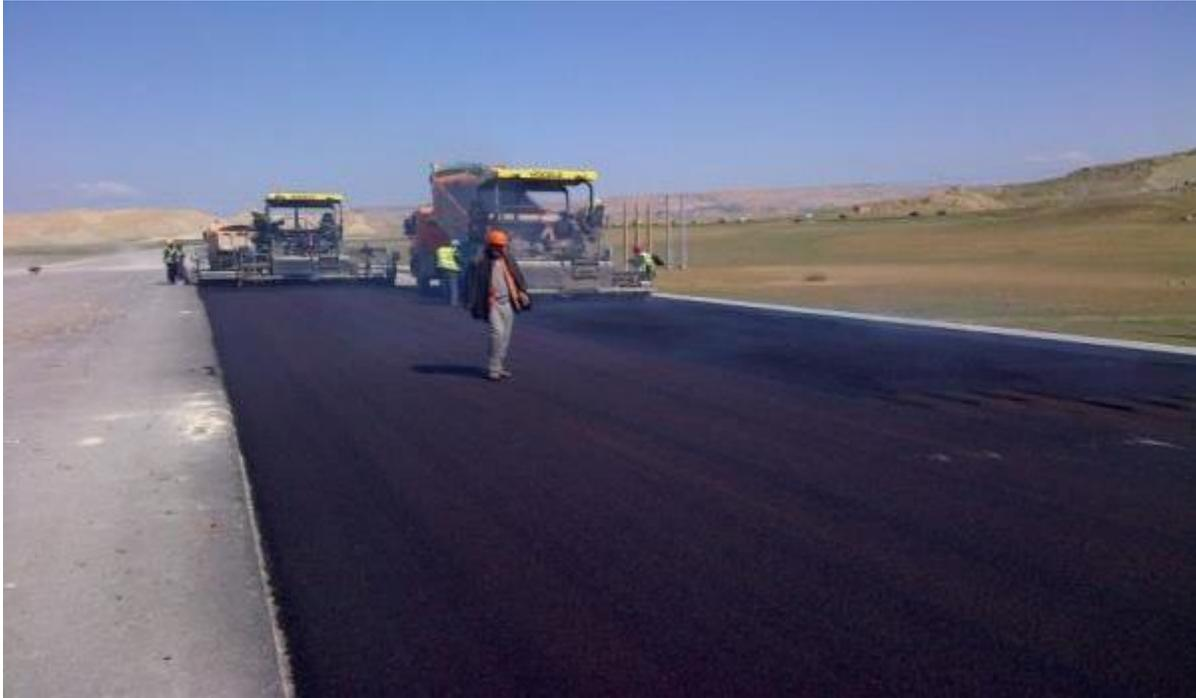
Fig. 8. EME2 and BBME with Superplast asphalt concrete paved in Northern Africa.
